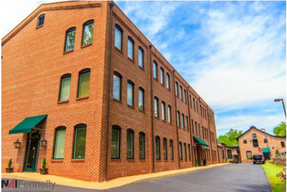
Building B; Rear/Side View
