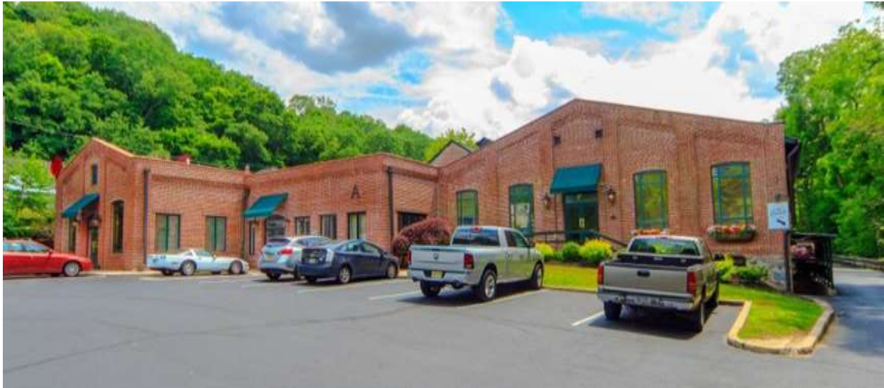
Building A; Front Exterior
