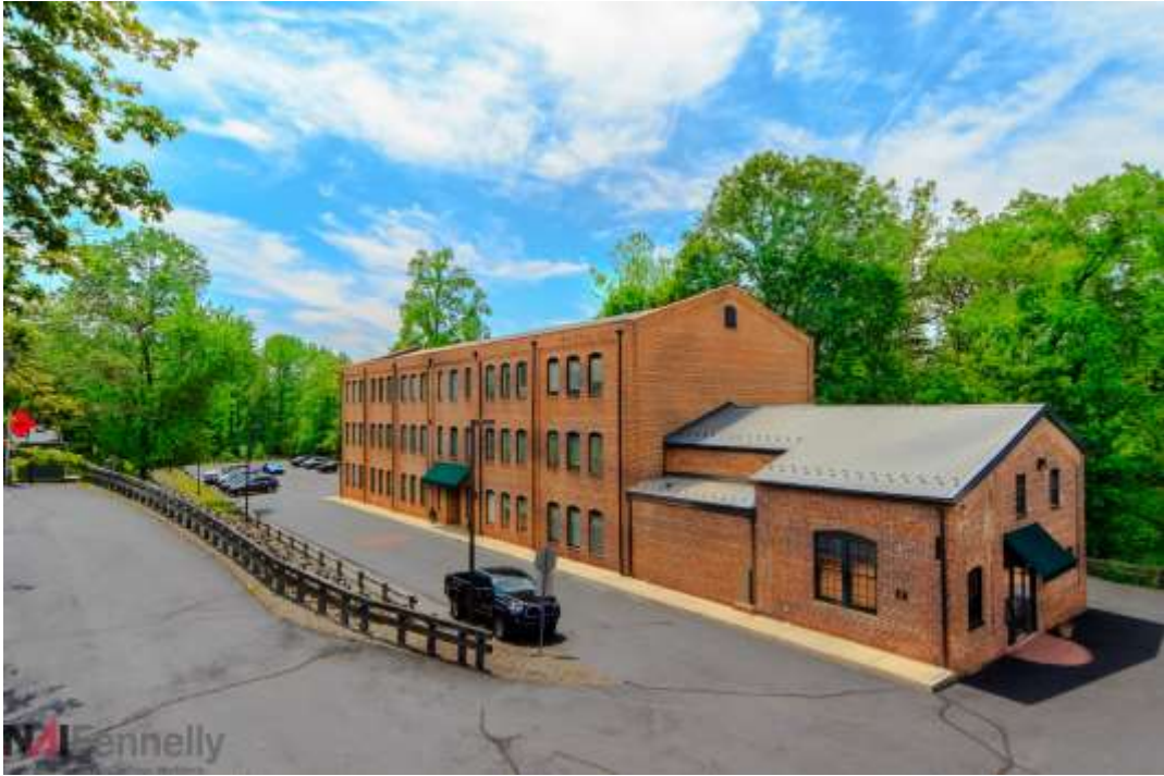
Building B; Front/ Side View
