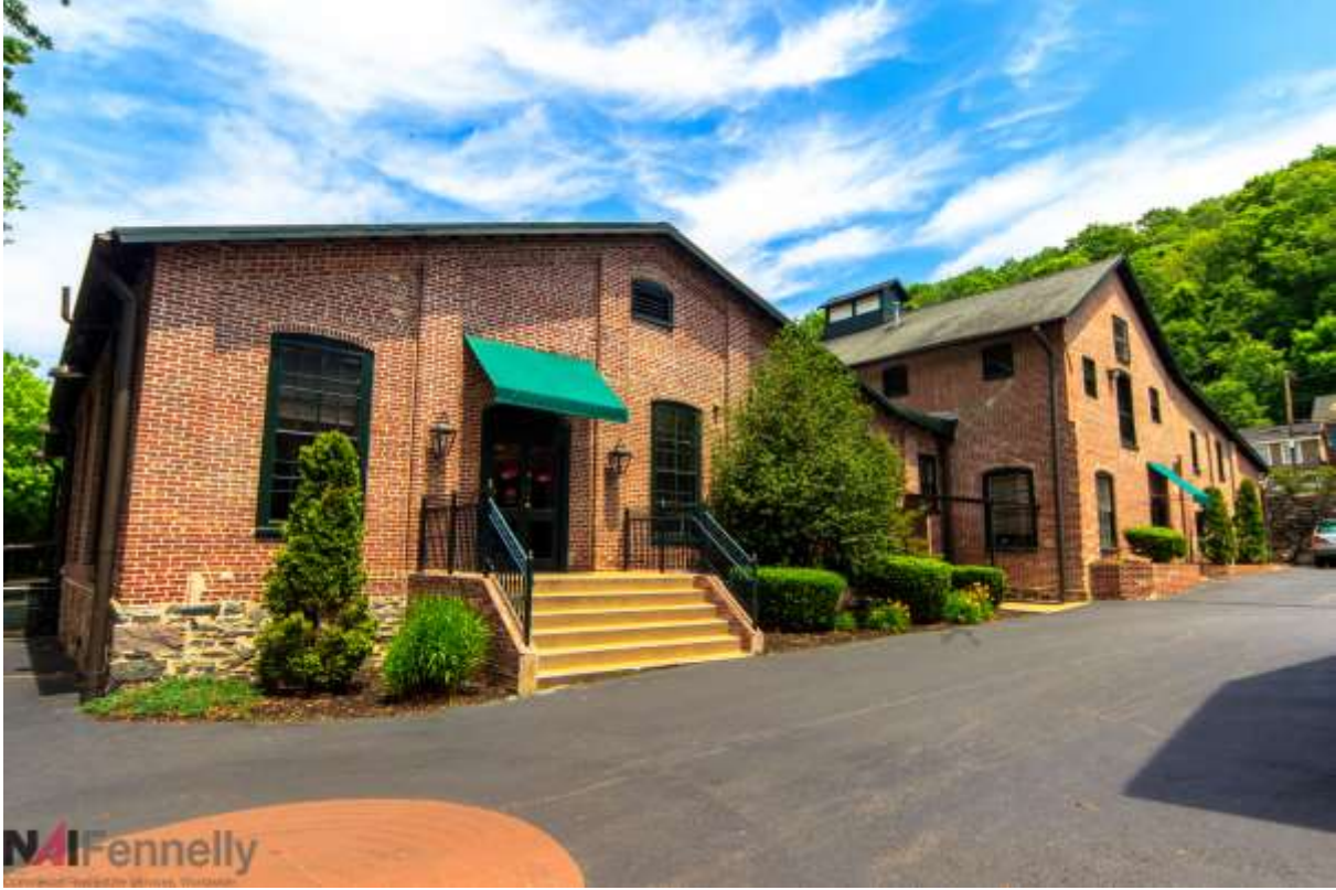
Building A; Rear Exterior View
