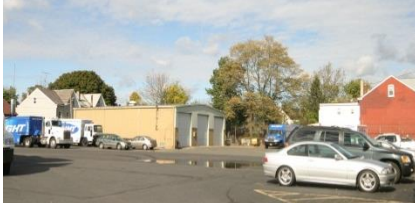
Repair Facility, Bldg. 4
