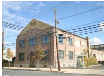
Two Story Office, 14,450 SF
