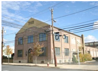
Two Story Office, 14,450 SF
